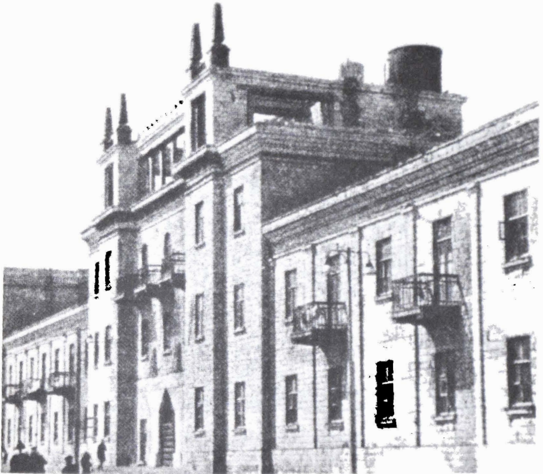
FIGURE 16.19 Apartment house in Krasnovodsk, Turkmenistan.
