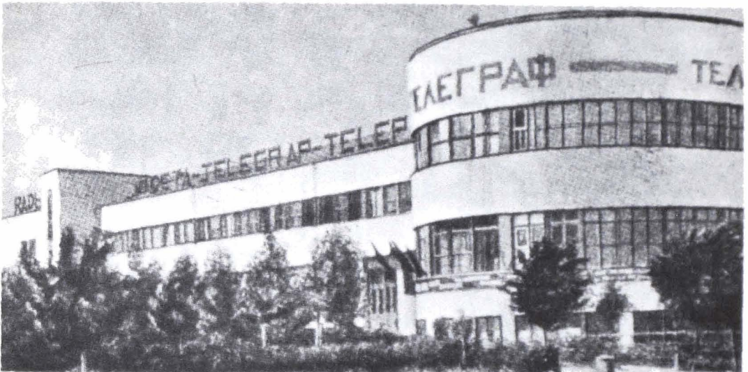
FIGURE 16.12 Alma Ata telegraph office building.
